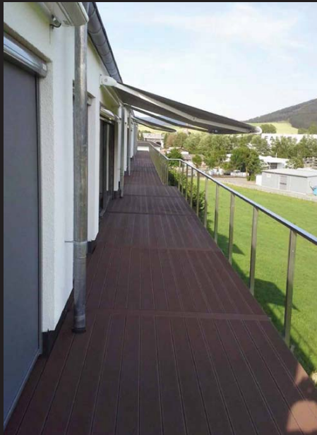
APARTMENTS | SCHMALLEMBERG | GERMANY balcony area
