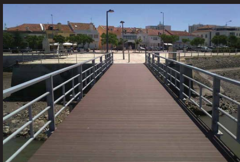
PEDESTRIAN BRIDGE | MOITA | PORTUGAL bridge area
