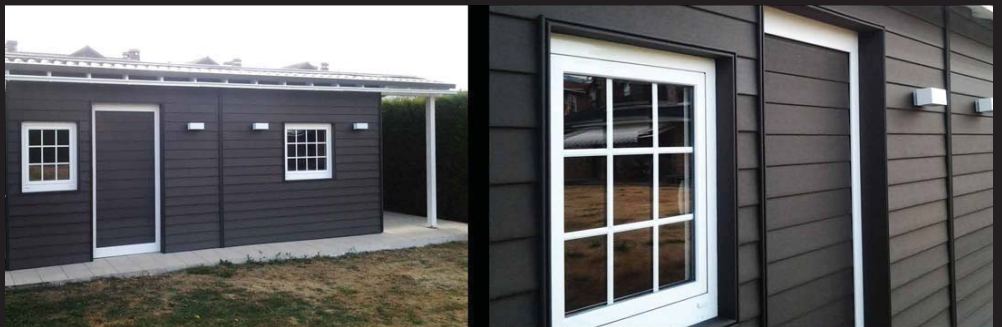
PRIVATE HOUSE | PAMPLONA | SPAIN house cladding
