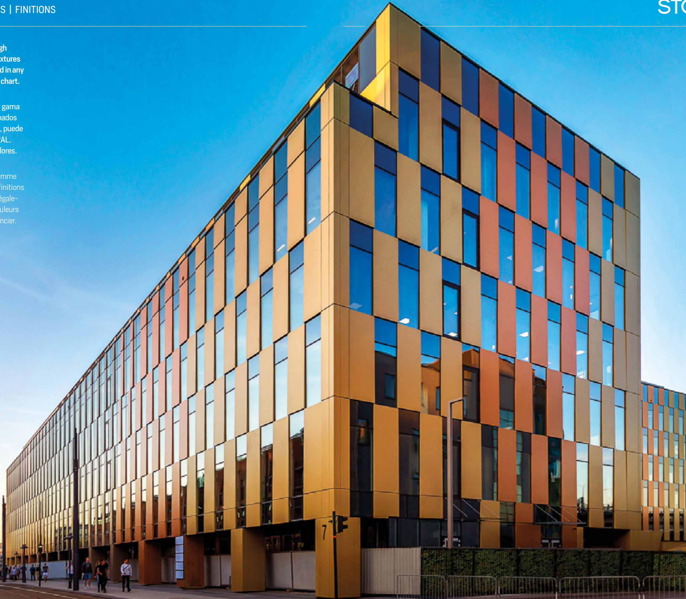
HIGH FIVE OFFICE BUILDING Krakow, Poland
